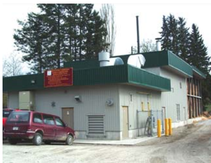
The biomass heat plant of Revelstoke's district heating system.
