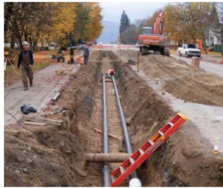
Laying district heating hot water pipes in the City of Revelstoke.
