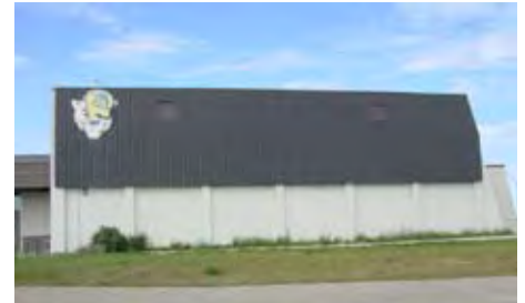
Solar wall on Dr. Kearney Junior Secondary School, Fort St. John – one of 3 solar walls in the school district, all working well, highly recommended by the school district, especially for new buildings.
