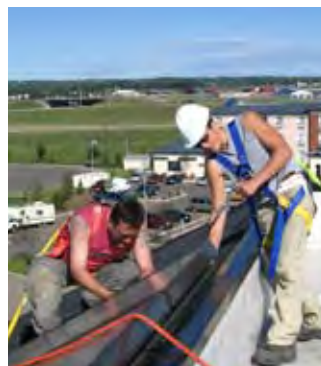
Installing solar hot water panels.
