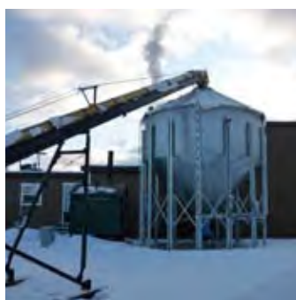
Baldy Hughes fuel silo.
