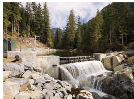
The intake and weir at the Furry Creek run-of-river power project. Source: Independent Power Producers Association of BC
