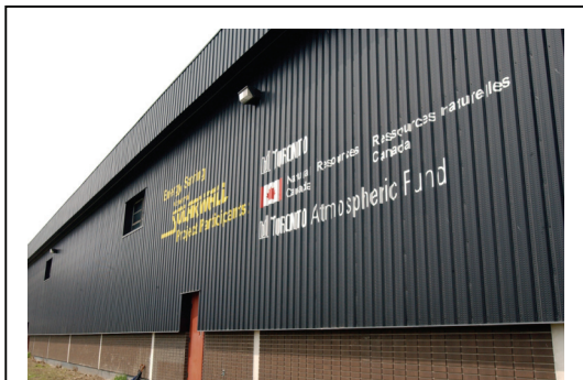
Energy saving Conserval SolarWall on the City of Toronto Vehicle Maintenance Garage. The south wall of the building is covered with 613 square metres of solar cladding. The system has reduced heating costs, enhanced indoor air quality and improved the overall appearance of the building.
