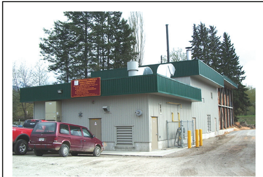
Revelstoke biomass district heating plant Source: Revelstoke Community Energy Corporation
