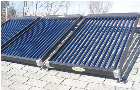
Evacuated tubes are commonly used in commercial facilities
