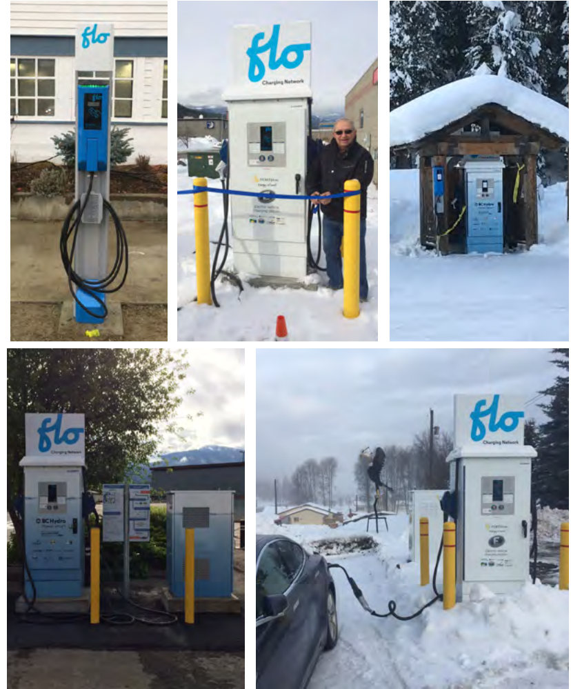
Clockwise from top left: A Level 2 pedestal charger; Castlegar Mayor, Lawrence Chernoff opening the FortisBC-owned DCFC in Castlegar; The BC Hydro-owned DCFC and Level 2 kiosk in Glacier National Park; DCFC in Greenwood, a key stop for travel between the Okanagan and the Kootenays; the DCFC in Sparwood.
