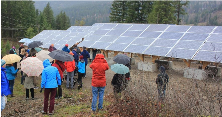
Figure 12 Nelson Solar Garden
